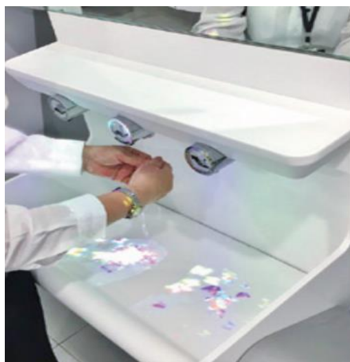
Figure 5.4 “One-stop” Hand-washing and Hand-dryer in One Basin
